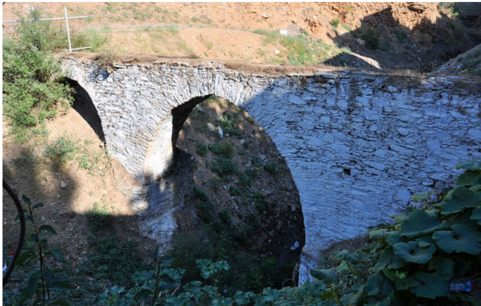
Fig. 7 Back View of Yahudi Deresi Bridge
