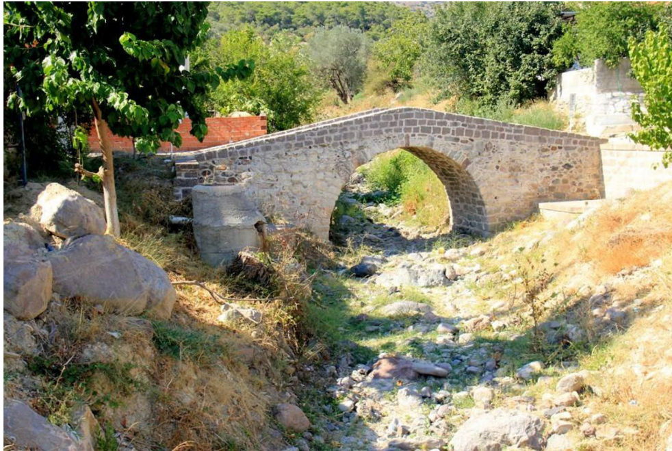
Fig. 4 Recent View of the Ignedere Bridge
