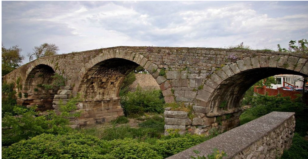
Fig. 2 Front View of Uc Kemer Bridge
