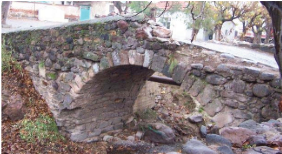
Fig. 5 Previous View of Ignedere Bridge before restoration
