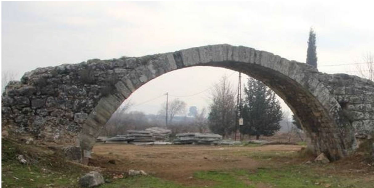
Fig. 8 Front View of Sarikemer Stone Bridge
