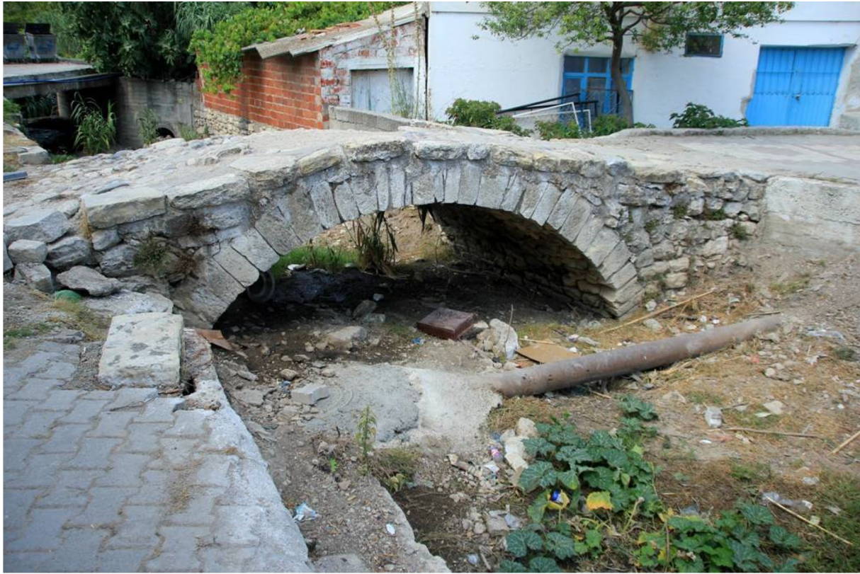
Fig. 10 View of Ozbek Village Bridge
