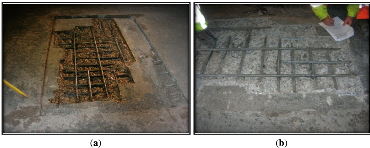
Figure 13. (a) Area of moisture damage (b) replaced with new rebars [37].
