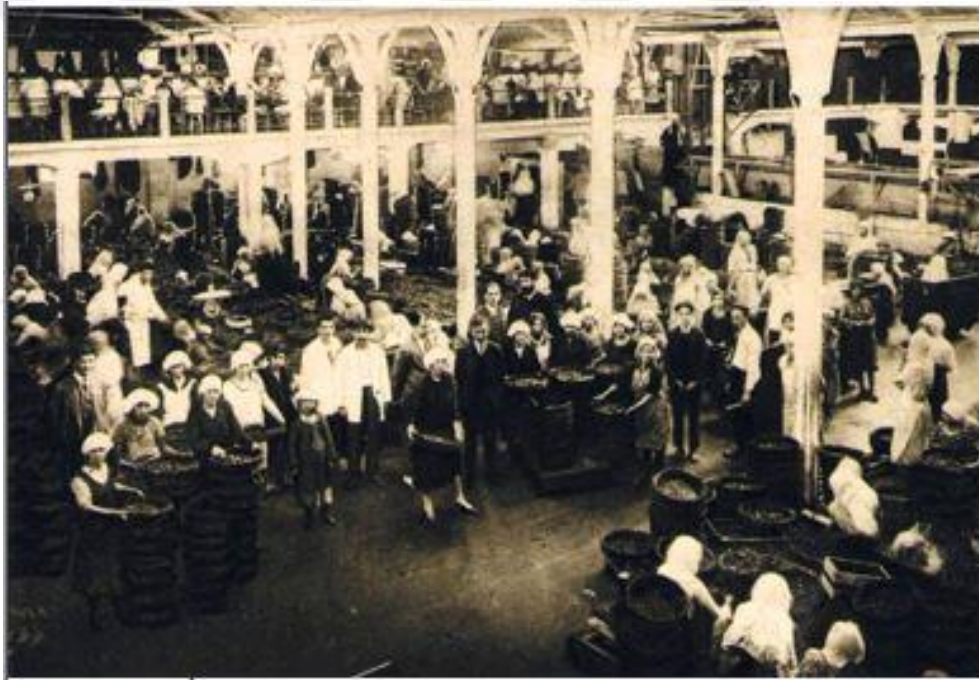
Figure 17: An example of an interior view of a fig han -courtyard plan scheme (Source: APIKAM, 2020)
