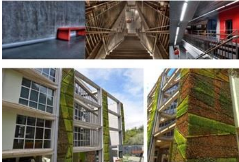
Figure 47. The FFAD building of Izmir University of Economics (Source: Arkiv, 2021; Google image, 2021)
