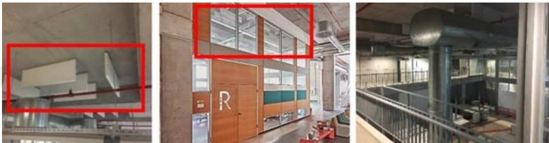
Figure 74. The recessed ceiling as a habitable poché for the suspended acoustic panels (Photos by: Seyedalipour, 2020)
