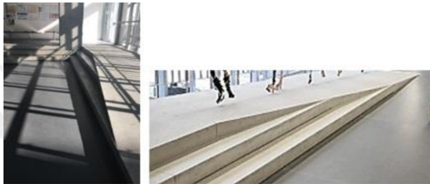
Figure 60. Angular relationship between the ramp and the stairs (Photos by: Seyedalipour, 2020)
