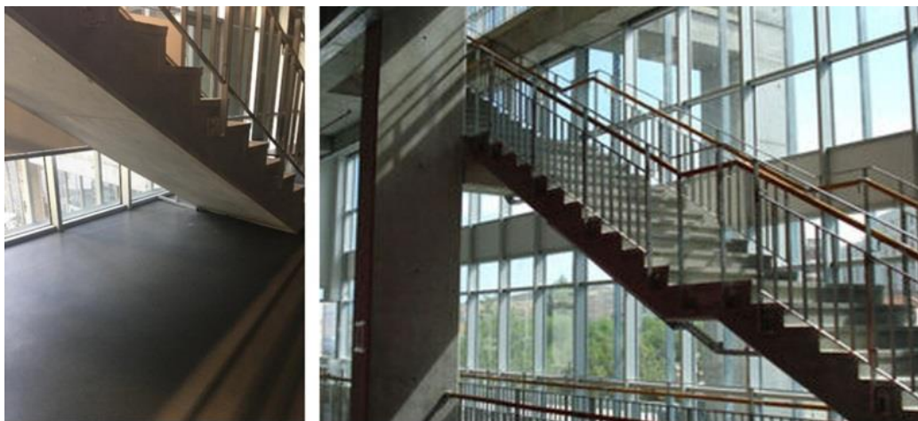
Figure 87. The triangular shape between the floor and the staircase (Source: Google image, 2020)
