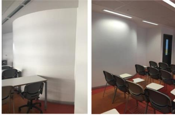
Figure 82. The protrusion of walls in the classrooms (Photos by: Seyedalipour, 2020)
