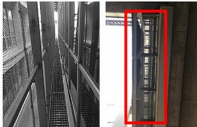
Figure 57. The gap between the double-skin façade as the second type of negative space (Photos by: Seyedalipour, 2020)
