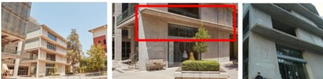
Figure 76. The protrusion of the concrete slabs as a habitable poché (Photos by: Seyedalipour, 2020)
