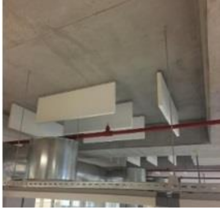
Figure 58. The recessed ceiling as a habitable poché for the suspended acoustic panels (Photo by: Seyedalipour, 2020)
