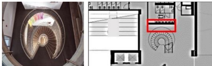
Figure 66. The gap between the restroom wall and the staircase (Photo by: Seyedalipour, 2020)
