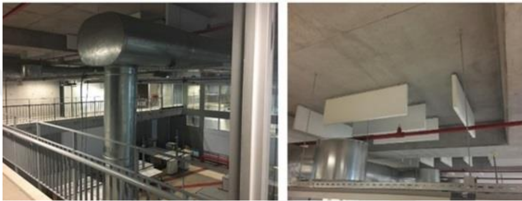
Figure 88. The recessed ceiling as a habitable poché for the suspended acoustic panels (Photos by: Seyedalipour, 2020)
