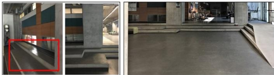
Figure 91. Continuity of the stairs and the ramp (Photos by: Seyedalipour, 2020)
