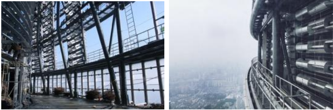
Figure 52. Wind Turbines of Shanghai Tower. (Source: left; Hu, 2022 right; The Architectural Review, 2015)
