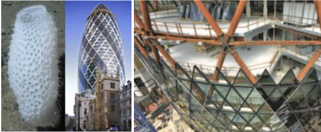
Figure 40. Left ;Venus Basket Sponge Right; A structural node on the façade of 30st Mary Axe.(Source: Nkandu and Alibaba, 2018)
