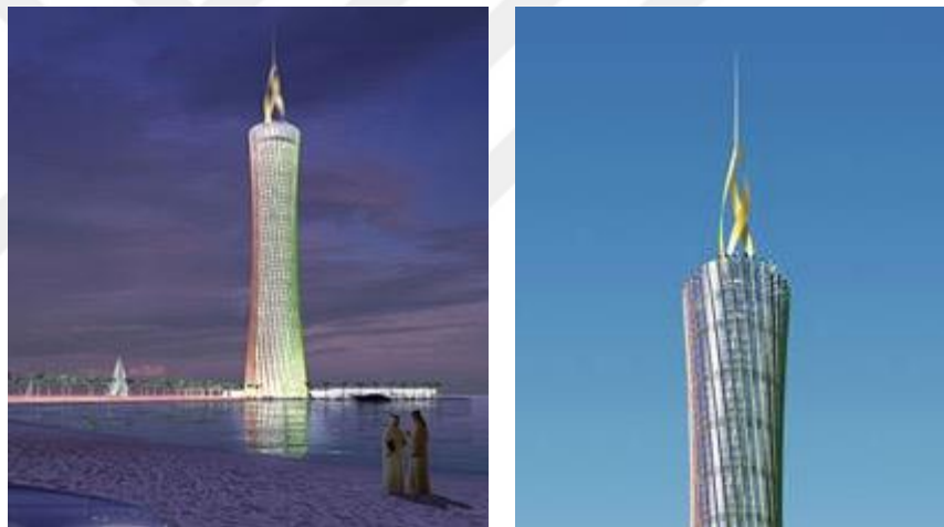
Figure 25. Burj al-Taqa in Dubai. Right; the wind tribunes at top. (Source: Design Build Network, 2008)
