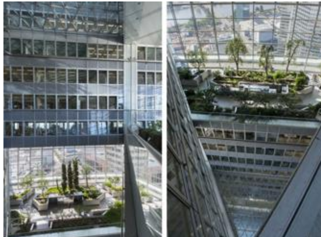
Figure 49. Commerzbank sky garden and atrium acting as ventilation chimney. (Source: Lotfabadi, 2015)
