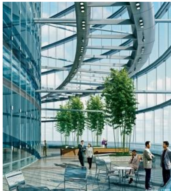
Figure 54. Exterior curtain wall of Shanghai Tower (Curtain Wall A) and an interior curtain wall (Curtain Wall B)—with a tapering atrium in between. (Source: left; Gu, 2015 right; CTBUH)
