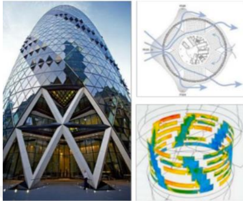
Figure 43. 30st Mary Axe ventilation strategies. Left: the blinds on the facades intercept solar energy by a 15% solar transmission rate. Right-top: the natural ventilation. Right-bottom: The wind flow. (Source: Küçük and Arslan, 2020)
