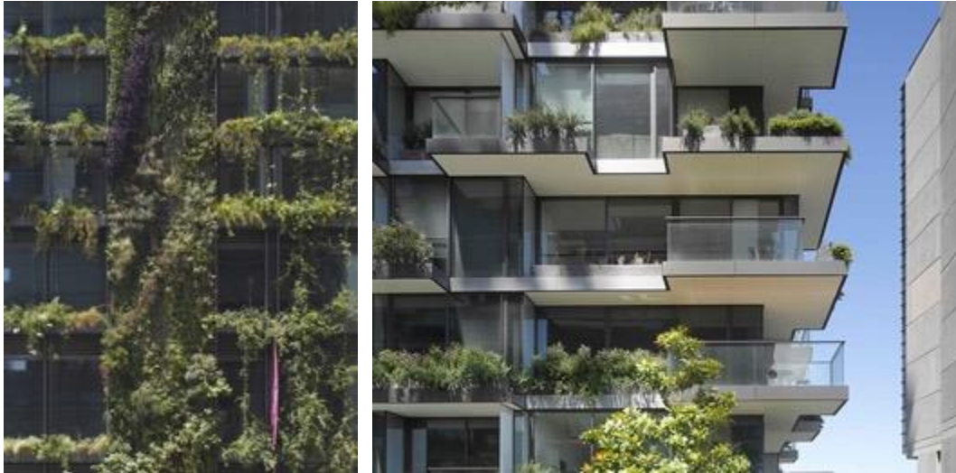
Figure 30. One Central Park façade. Hydroponics Wall –Vertical Gardens by Jason A. Dibbs. Right; Polyethylene planter boxes on the façade to provide organic shade. (Source: AJN, 2010)
