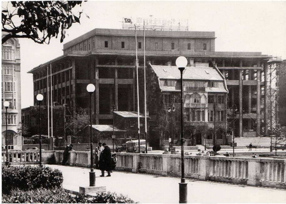
Figure 19. The carcass of the opera house that has stood for a long time in Taksim square (Source: Can, 2014)
