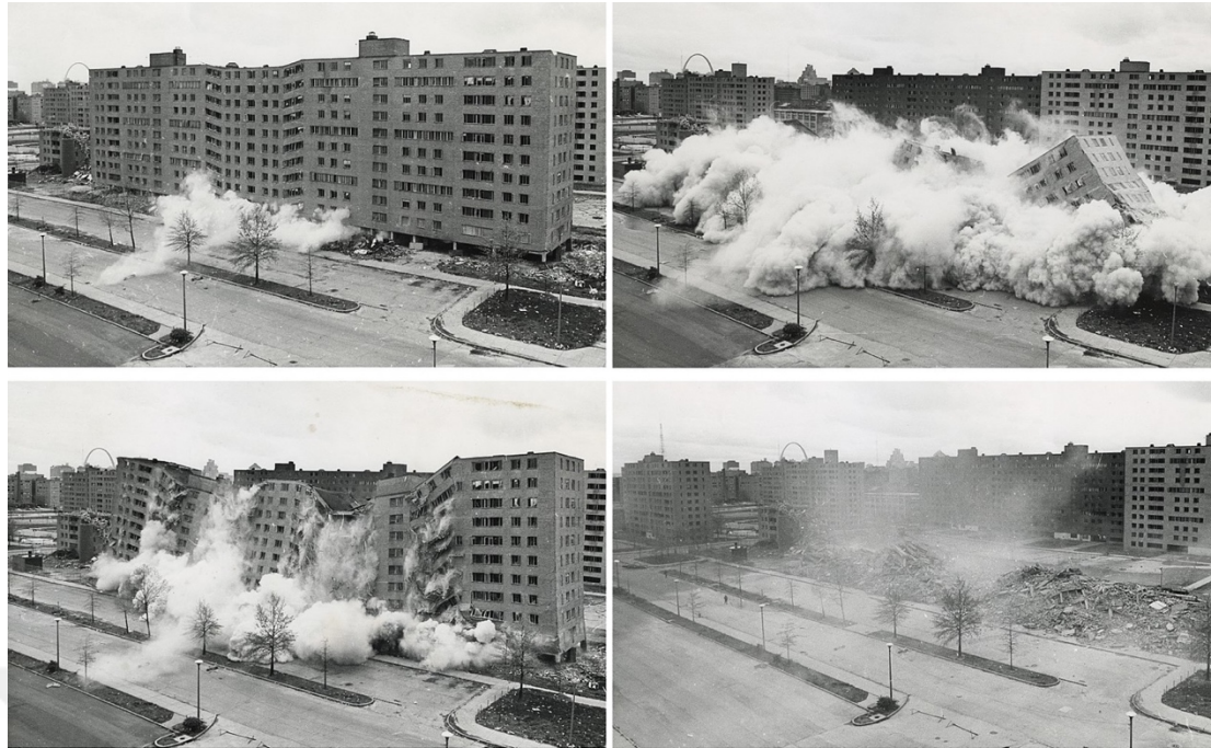
Figure 1. Demolition of a Pruitt-Igoe Building (Source: Fiederer, 2017)
