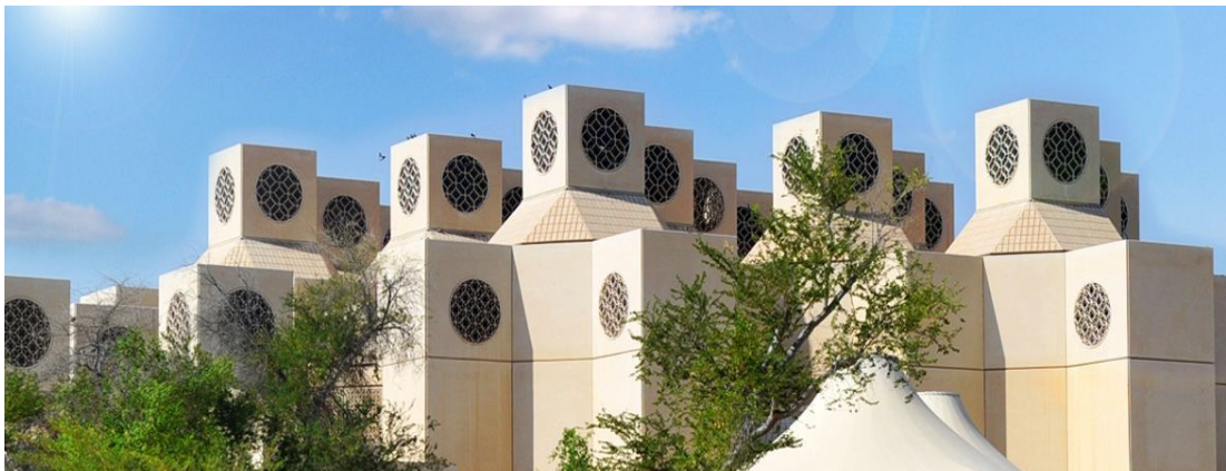
Figure 130. New type of windcatcher used in the university of Qatar. (Source: Baldwin, 2021)
