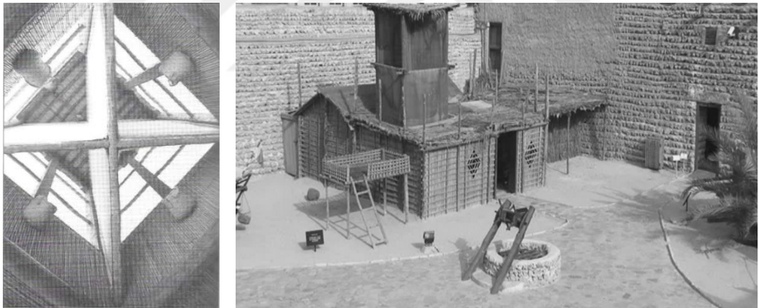
Figure 65. The interior view of the palm frond wind tower (left), the courtyard view (right) in the UAE (Source: Hawker, 2008, p 60).
