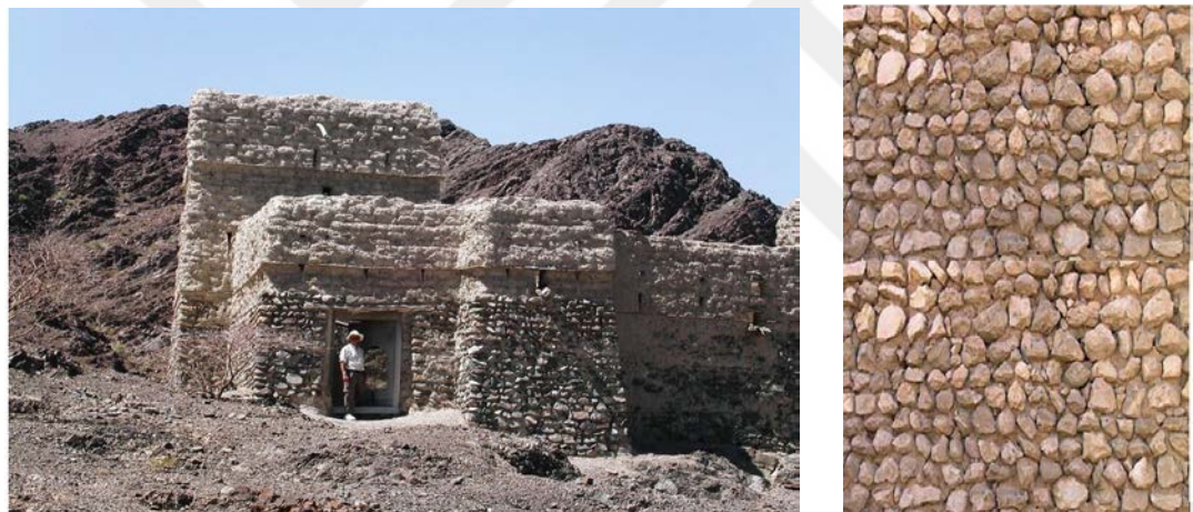
Figure 45. Shows the common stone houses near the mountain of the coast of UAE and Oman (left) (Source: Patternson, n.d.) and (right) shows the traditional placement of the layers. (Source: Lockerbie, 2021)
