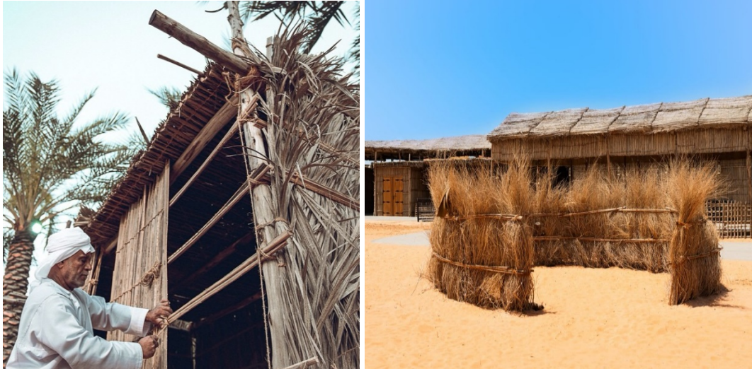
Figure 42. the arish palm frond house, (left) showing the local building it and (right) a sample structure in the, Sharjah UAE. (Source: weebly.com)
