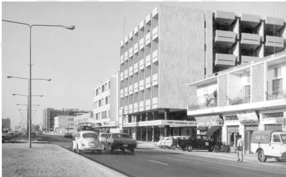
Figure 29. A view of the First National City Bank on Sharjah, UAE. (Source: EL-Tohamy, 2021)
