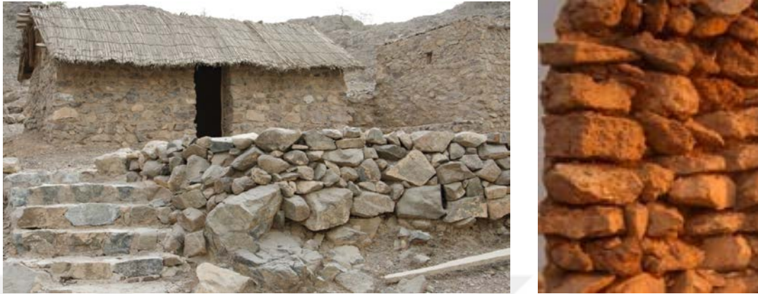
Figure 44. An example from UAE stone house with palm frond roofing (left) (Source: Anon., 2007) and the typical stone layer (right) (Source: Lockerbie, 2021).
