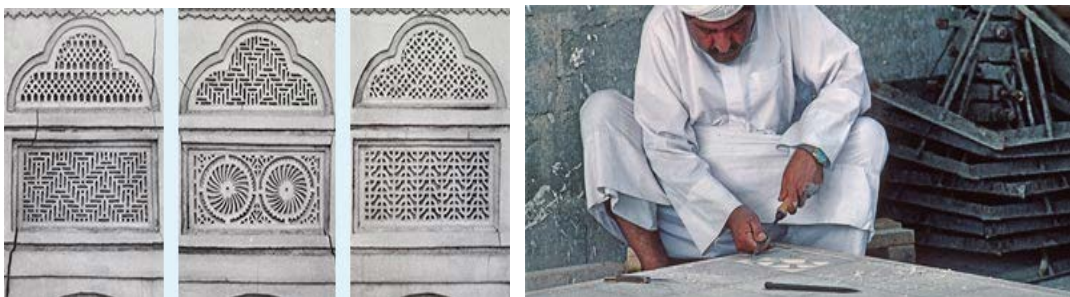
Figure 39. (left) the Nuqsh plaster panels and (right) the carving method where the mason carving pattern with a knife. (Source: Lockerbie, 2021)
