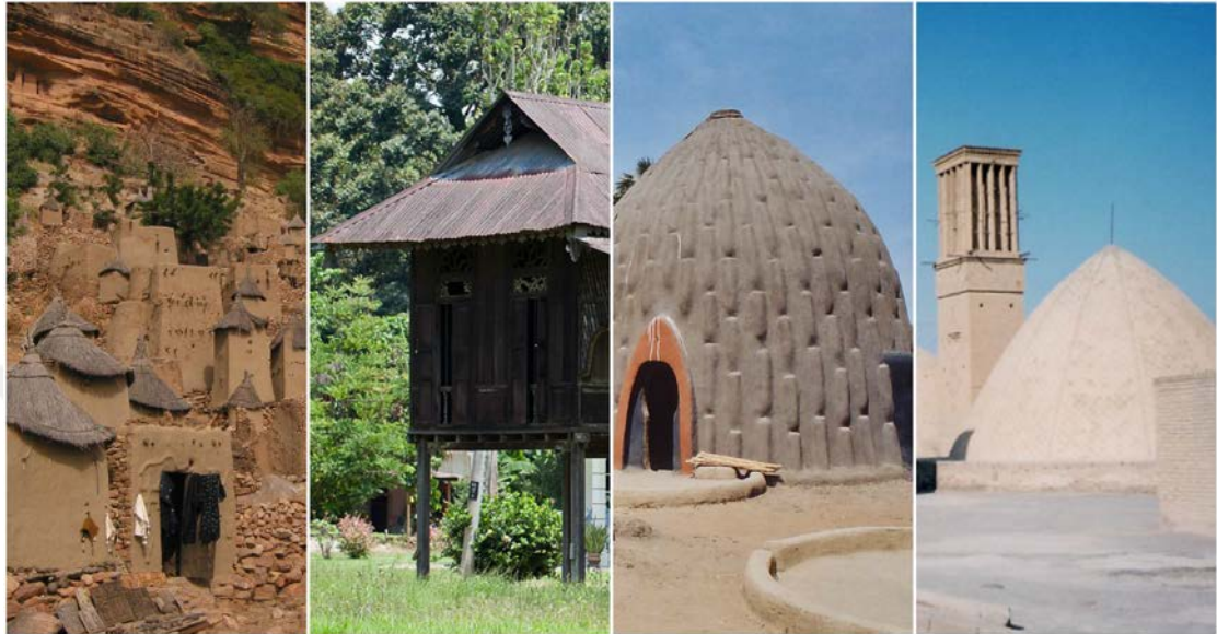
Figure 2. Vernacular architecture from different regions (from left to right) Cliff of Bandiagara, Mali, Malay Houses, Malaysia and Singapore, Mugsum Mud Huts, Cameroon, Ab-anbar, Iran (Source: archdaily, 2020)
