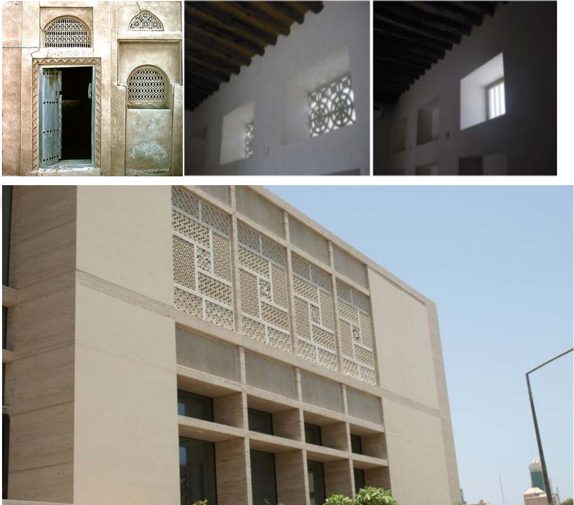
Figure 125. Shows the alternative window opening option with the privacy, as light enters through the perforation and also the view to the interior is minimized. Source: (Lockerbie, 2021) and the bottom shows a contemporary use of the nuqsh panel in Kuwait. (Source: Kassam, 2016)
