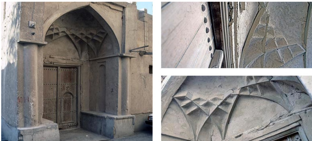
Figure 112: muqarnas used as a decorative element in the pedestrian entrance in Qatar. (Source: Lockerbie, 2021)
