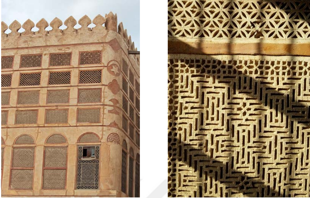
Figure 40. the plaster works example on the Siyaddi house, Bahrain. (Source: Zakharia, 2016)
