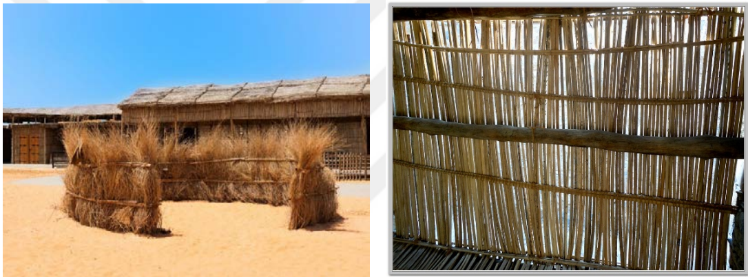
Figure 111. (left) example from Dubai shows a tradition arish structure and (right) shows the spacing to allow for the air to follow and keep the house cooler. (Source: Bayt, n.d)
