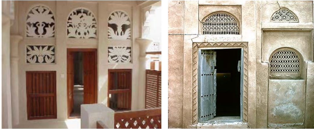
Figure 85. shows the example of Nuqoush Muftah upper openings provide natural ventilation and lighting (Source: Lockerbie, 2021)
