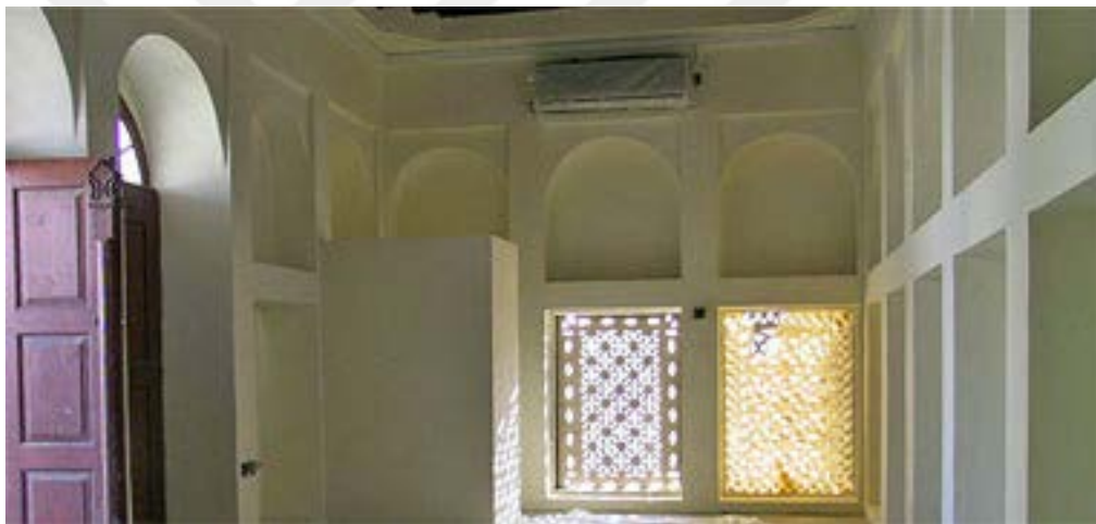
Figure 98. shows the diffusion of light into the room through the Nuqsh panels (Source: Lockerbie, 2021)
