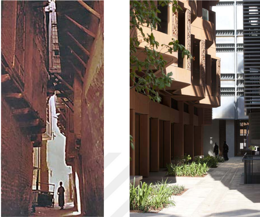
Figure 128. The mashrabiya over the sikkak narrow pathways left in the traditional Persian alleyways (left) (Source: Lockerbie, 2021) and the use of contemporary mashrabiya in the alleyway in Masdar project Abu Dhabi (right). (Source: Baldwin, 2021)
