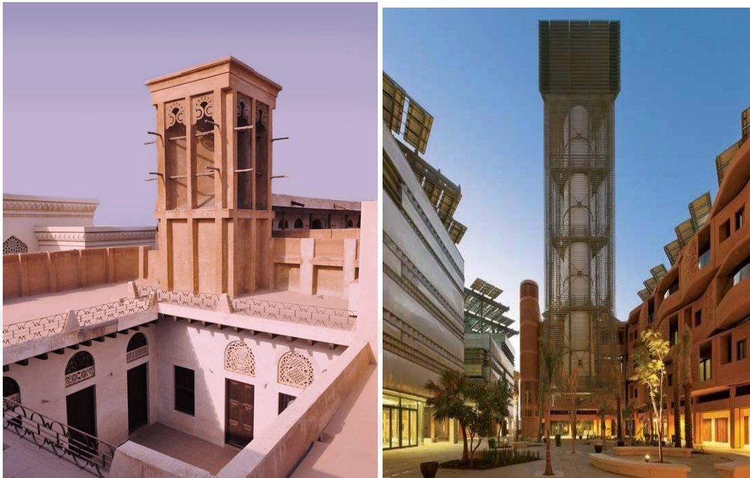
Figure 129 .(left) Shows the classic example of a wind tower as well the interior courtyard. and also, the openings above the doors and (right) a contemporary version of badgheer used in Masdar project Abu Dhabi. (Source: Baldwin, 2021)
