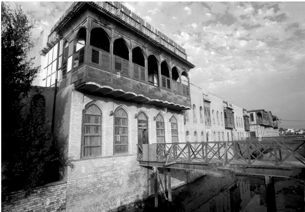
Figure 115. (top) an illustration of indirect view through the screen and (bottom) an example of these mashrabiya screens on balconies, Old city Basra, Iraq. (Source: Karban , et al., 2021)
