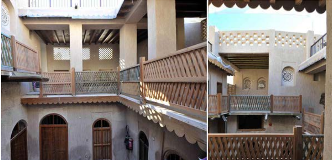
Figure 110. shows the wood work balustrade and doors, AL-Aqaili House, Deira, Dubai. (Source: weetas.com, n.d)
