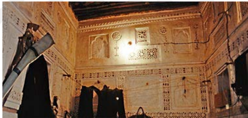
Figure 52. the use of the roof and interior of the Arab masonry housing. (Source: Lockerbie, 2021)
