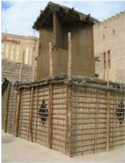
Figure 66. Wind towers constructed from palm frond in Abu Dhabi and Dubai (Source: Rashdan, Wael and, Vrushali, 2019)
