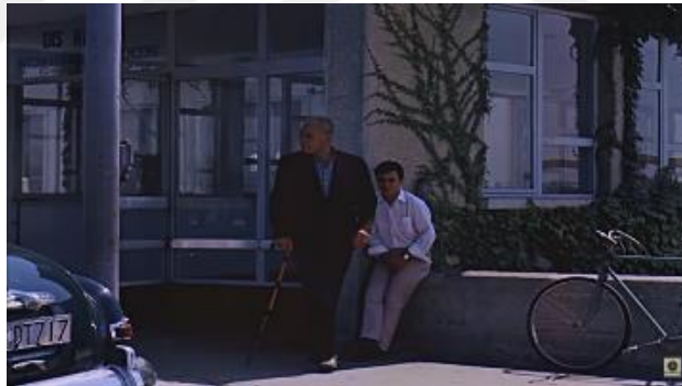
Figure 22: Main entrance of Yeşilköy Airport (Source: İnanoğlu, 1969)
