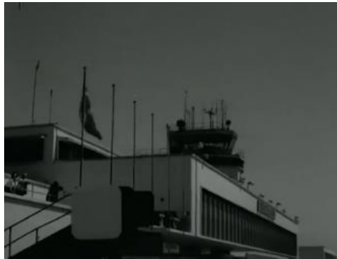
Figure 23: Yeşilköy Airport and control tower (Source: Saydam, 1965)
