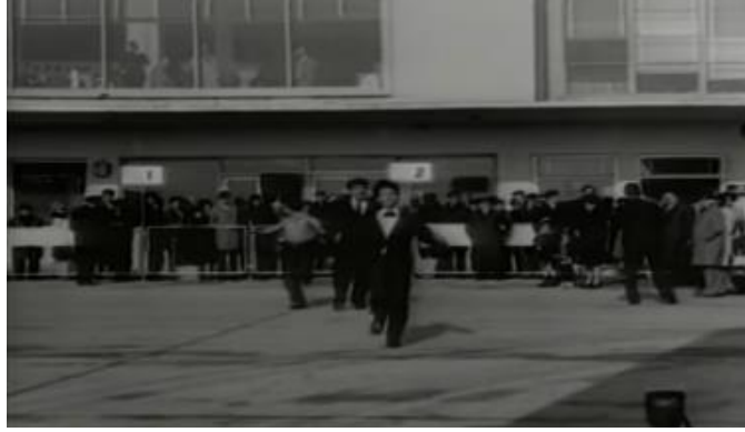
Figure 39: View façade of Yeşilköy Airport (Source: Seden, 1966)
