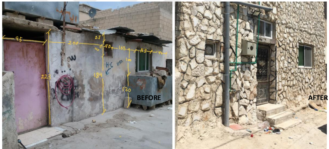
Figure 4.24: Exterior shot of the sample house unit before and after the rehabilitation
