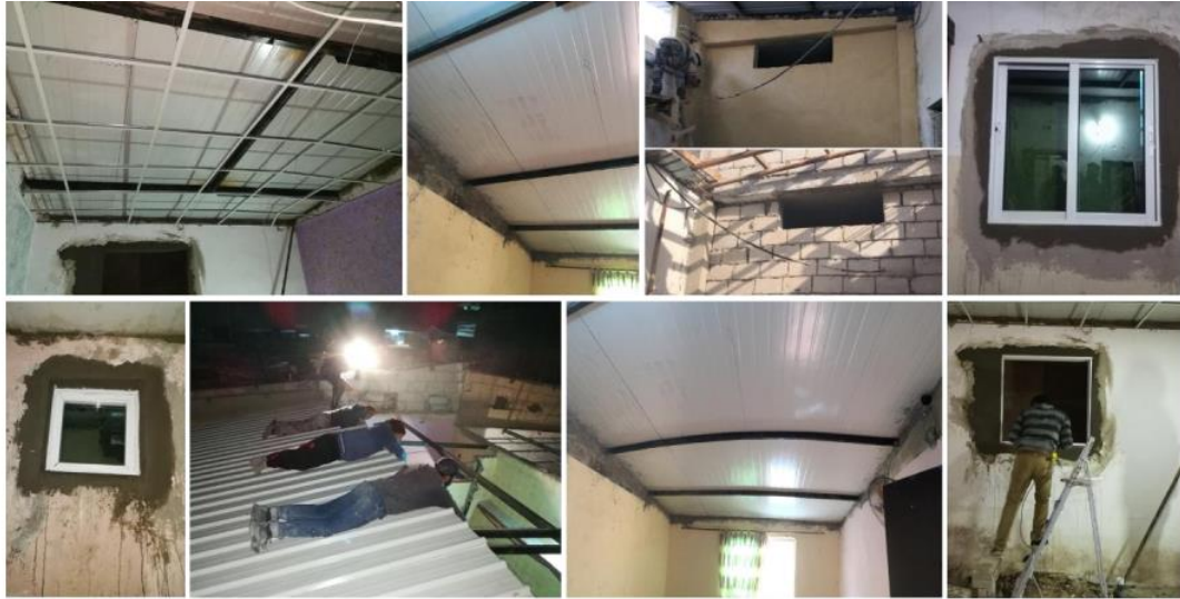
Figure 4.23: Images showing the first rehabilitation phase of the sample unit.
