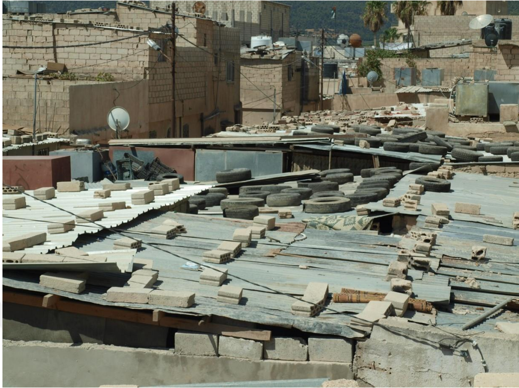
Figure 4.17: Bricks and car tires placed over the rooftops to stabilize it from the wind.
