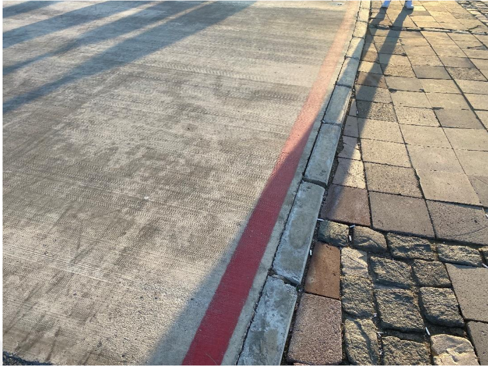
Figure 26. Pavement before arriving at Gündoğdu Square
