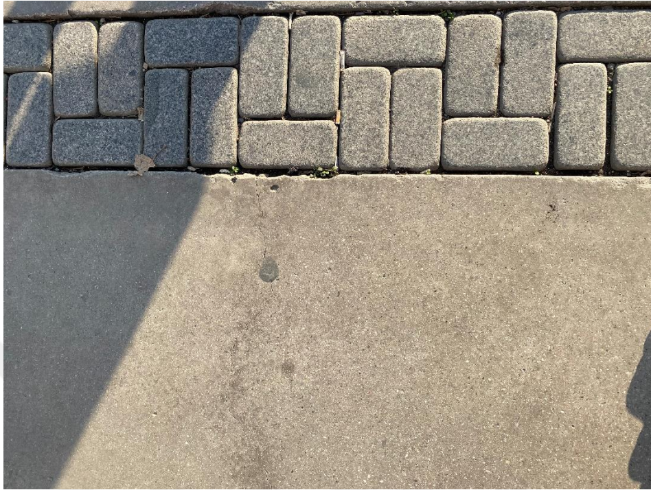
Figure 3. Pavement in Kıbrıs Şehitleri Street
