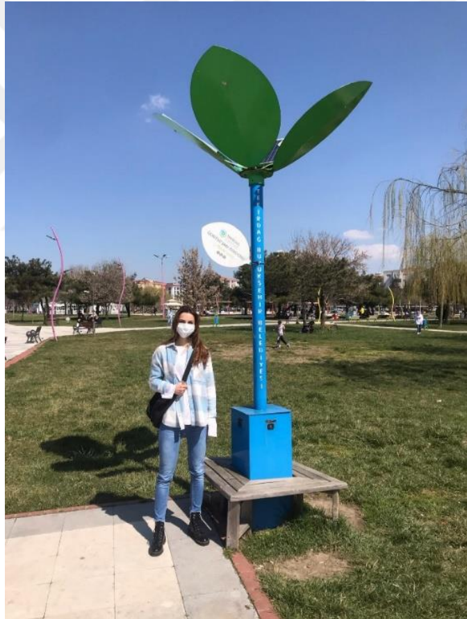
Figure 36. Solar charging station in Çorlu Republic Park.
