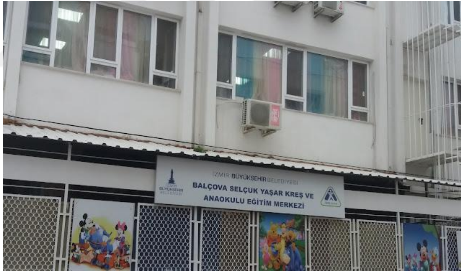
Figure 1: Exterior view of Balçova Selçuk Yaşar Nursery and Kindergarten Education Center. (Source: SuperRehber, 2022)
