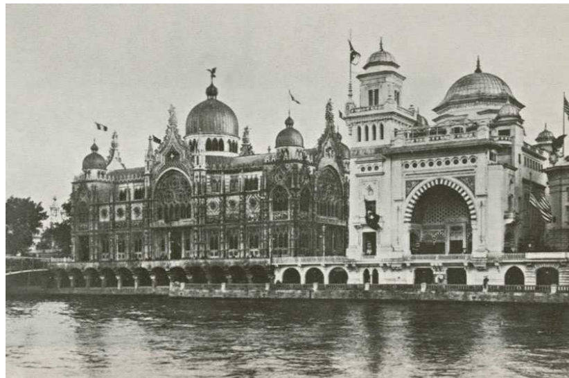
Figure 9. Rue des Nations, Ottoman pavilion to the right, Paris, 1900.
