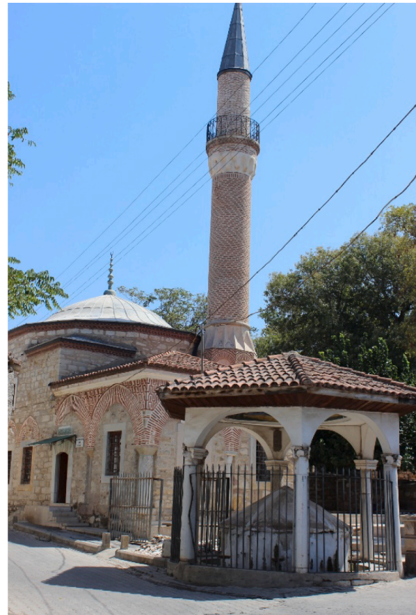
Fig. 5. Front View of case study 1 building.
