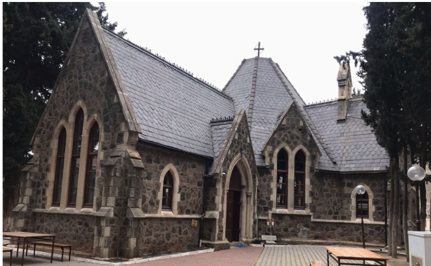
Fig. 7. Front View of case study 2 building.
