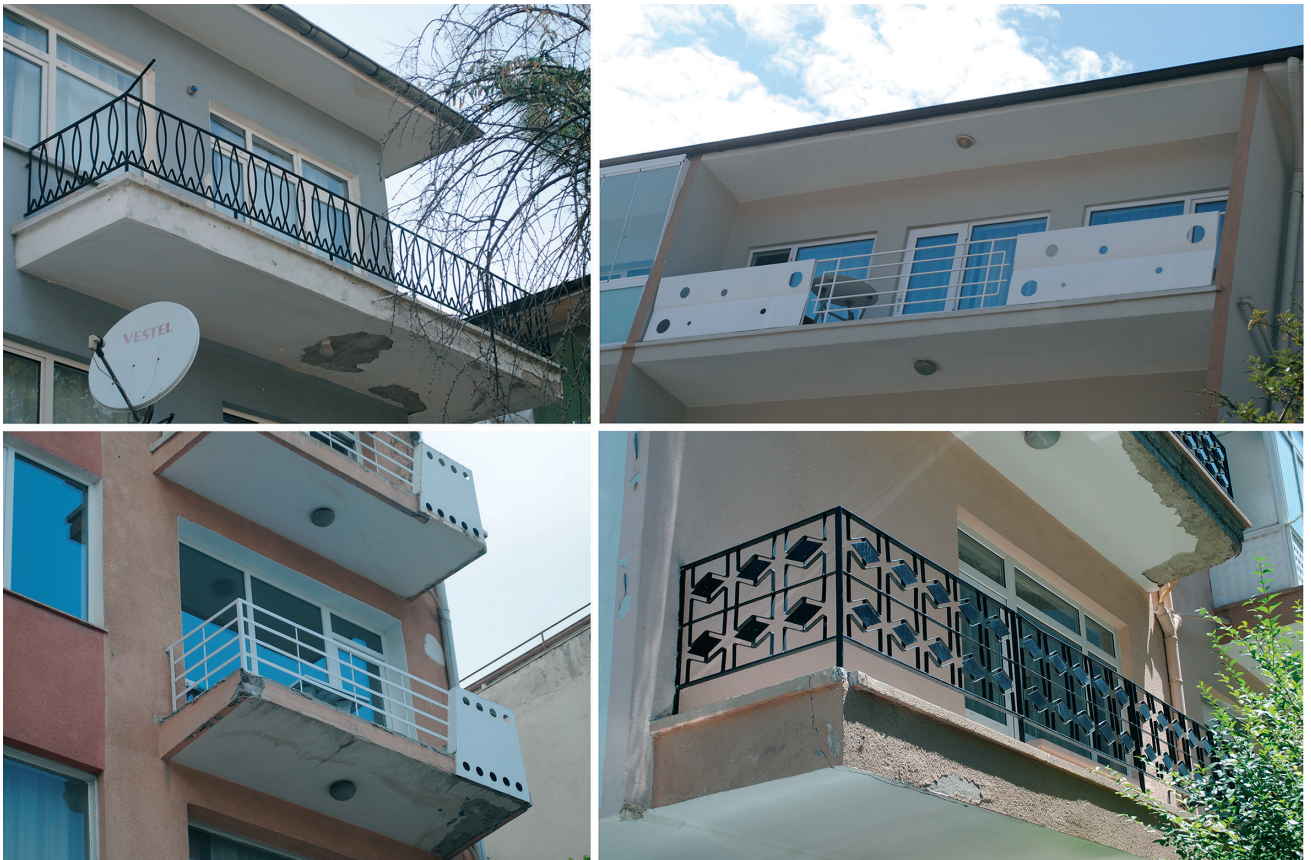
Figure 4. Balustrades from the research project illustrating authentic qualities (Tuna Ultav archive)
