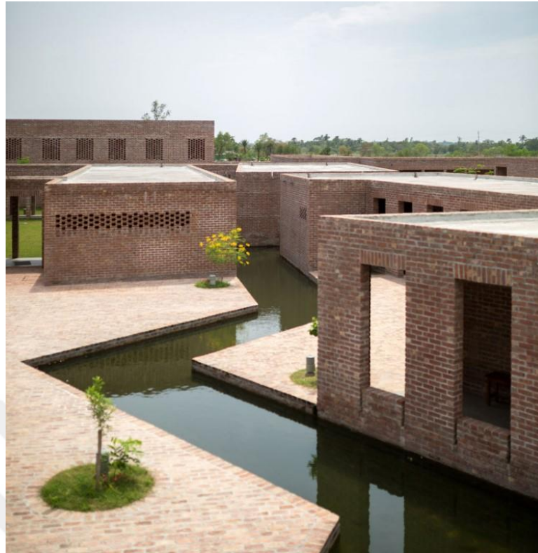
Figure 32. The canal that harvesting water (Source: archeyes.com, 2021)
