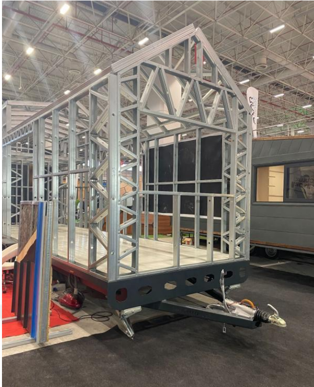
Figure 5. Steel structure in TINY HOME SHOW
