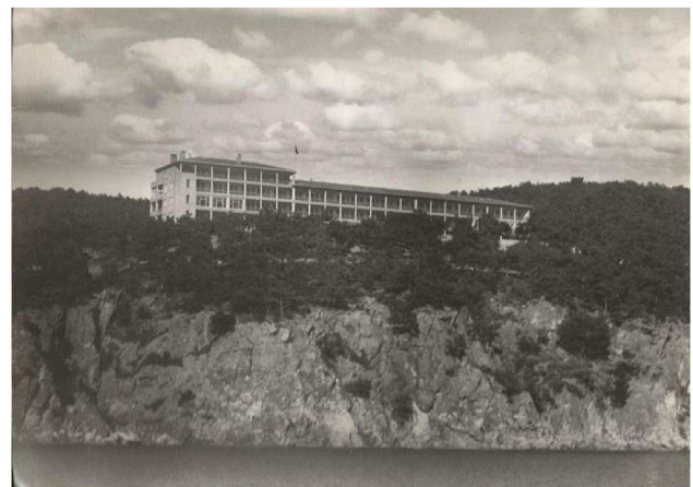
Fig. 25 The Block B of Heybeliada Sanatorium. Source: Courtesy of Gorbun Family archive.
