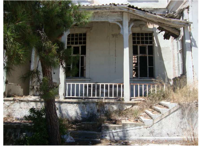
Fig. 13 The cure balcony of Pavilion A1. Source: Photograph by The Authors (2014).
