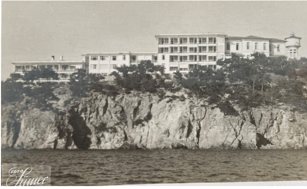
Fig. 2 Front/southern view of the entire Block A of Heybeliada Sanatorium (between 1939 and 1951). Source: The Authors' personal archive.
