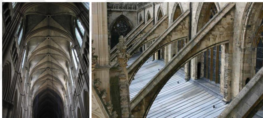
Figure 2a & 2b. Rib Vaults & Flying Buttresses (Source: https://en.wikipedia.org/ , 2023, https://www.thoughtco.com , 2019)
