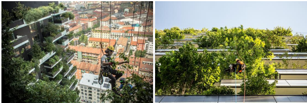
Figure 26a & 26b. Maintenance of Bosco Verticale (Source: https://www.archdaily.com/ )
