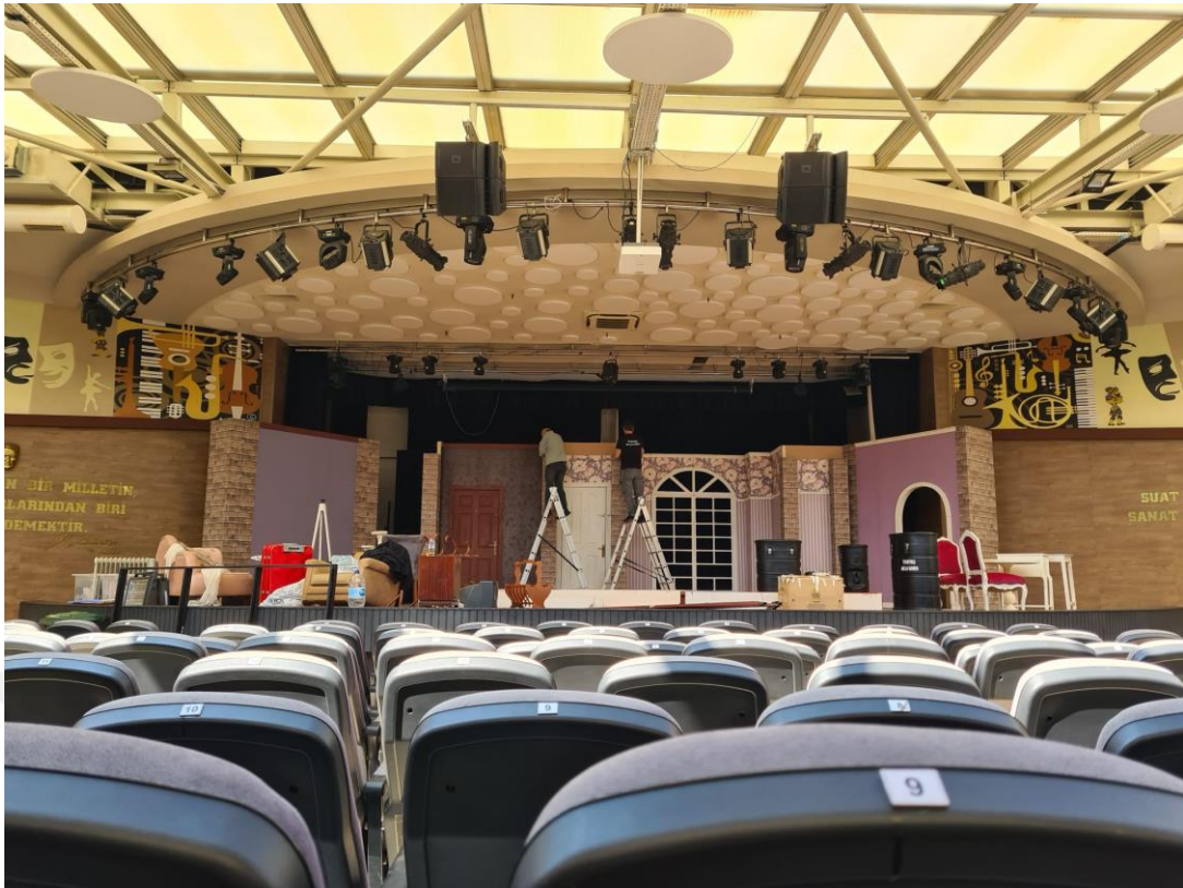
Figure 27. Installation of the Columns onto the Theatre Flats, 2023.
