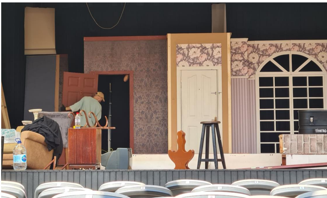
Figure 26. Installation of The Door into a Theatre Flat, 2023.
