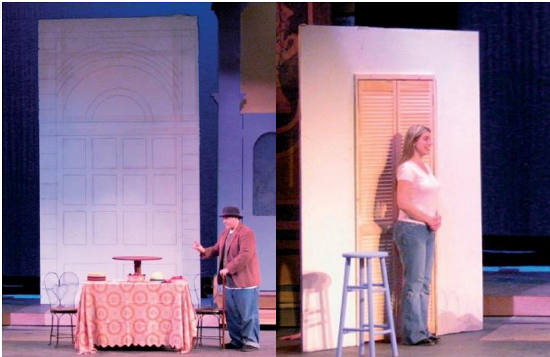
Figure 3. Examples for Soft-Cover Flat and Hard-Cover Flat (Source: Gloman and Napoli, 2007, pp. 5-6).
