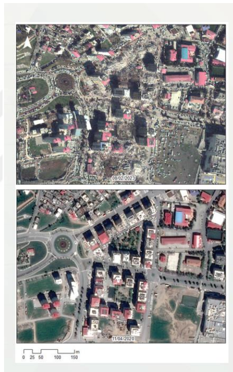
Figure 4. Satellite images of Kahramanmaraş center before and after the earthquake (Source: İTÜ, 2023, p. 54)
