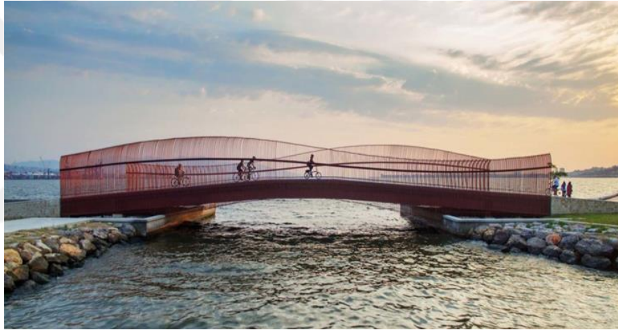
Figure 48. Bayraklı Pedestrian bridge (Source: Itez, 2020)
