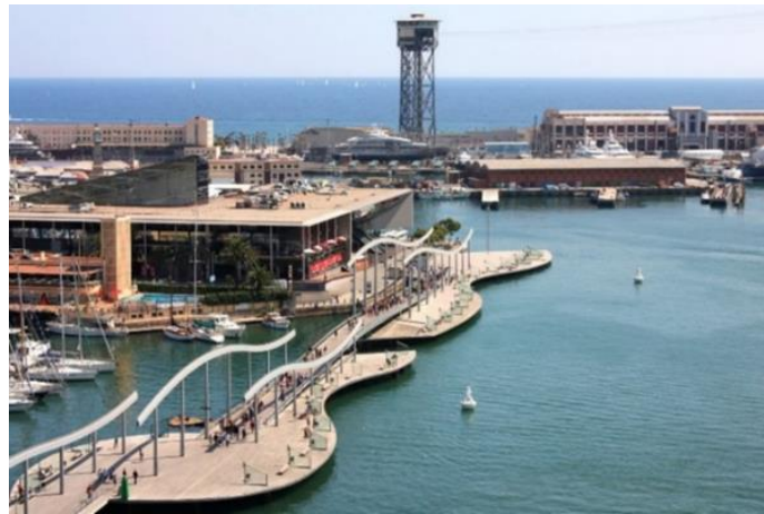
Figure 6. Port Vell's bridge in Barcelona (Source: hotels.com)
