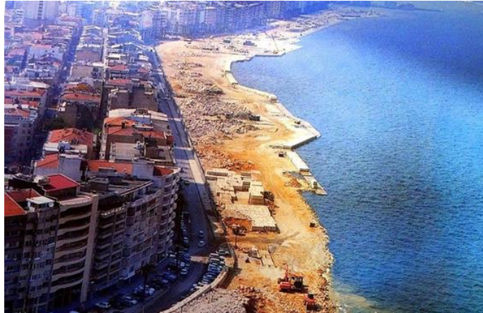
Figure 20. The land reclamation operations on the Kordon (Source: Izmirmag, 2016)
