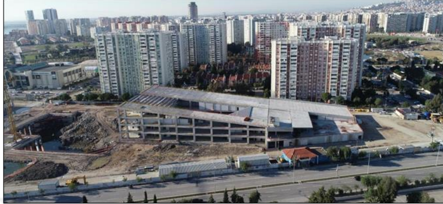
Figure 56. Final view of the construction of the Opera Center (Source: Karakoç, 2022)
