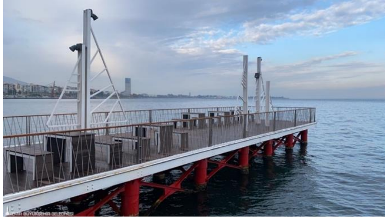
Figure 44. Pier on the shoreline (Source: Izmir Metropolitan Municipality, 2021)
