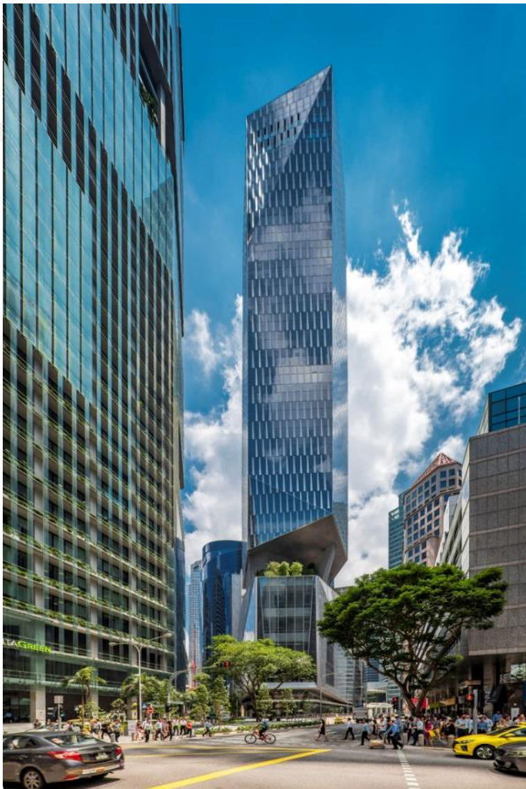
Figure 34. Robinson Tower Outside View (Source: Abdel, 2018)
