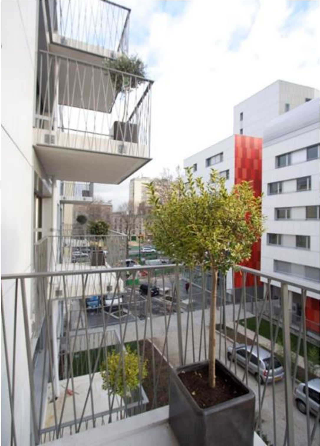
Figure 3. H&E Housing 1 (Source: Architecte, 2008)
