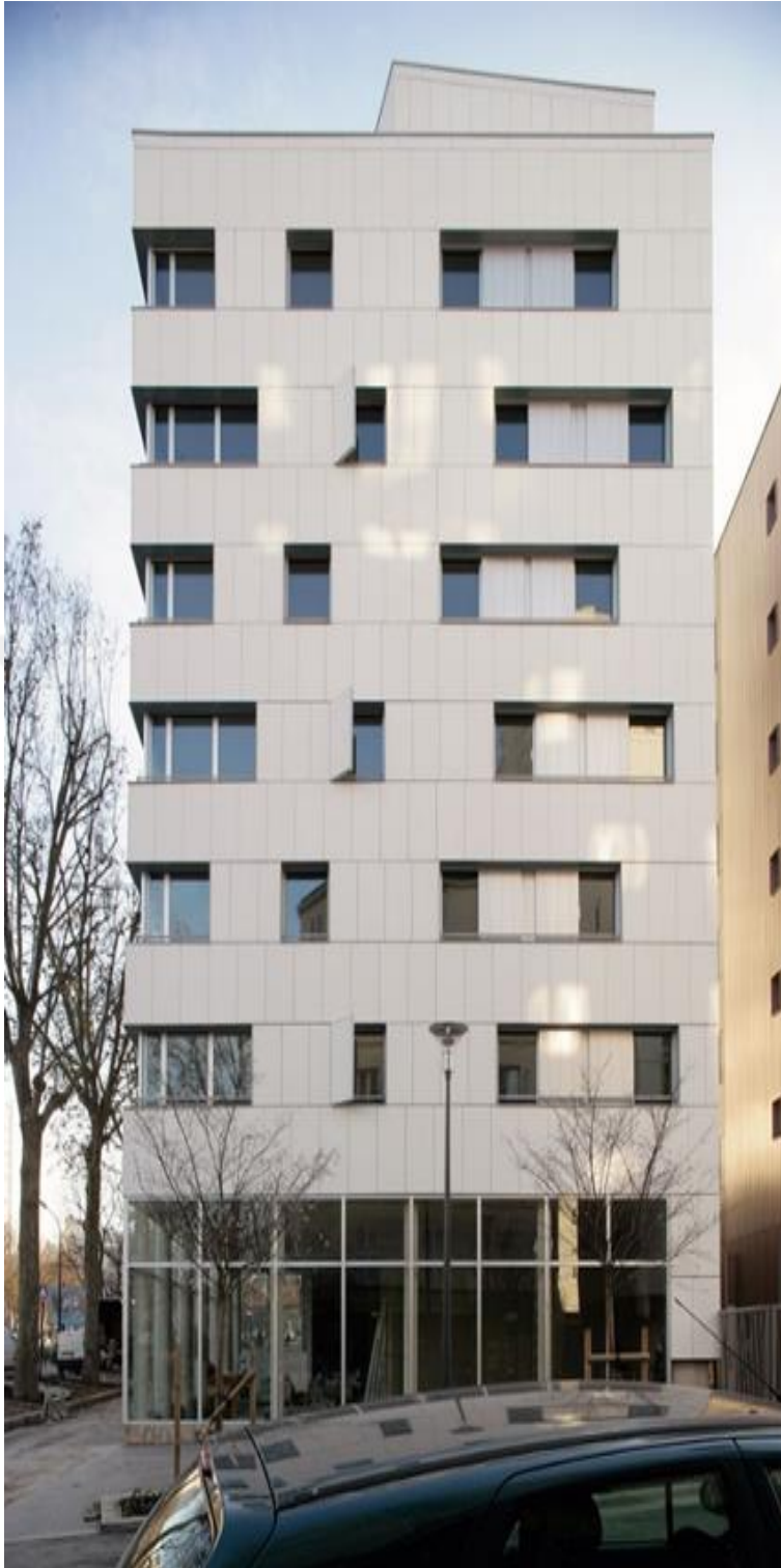
Figure 4. H&E Housing 2 (Source: Architecte, 2008)
