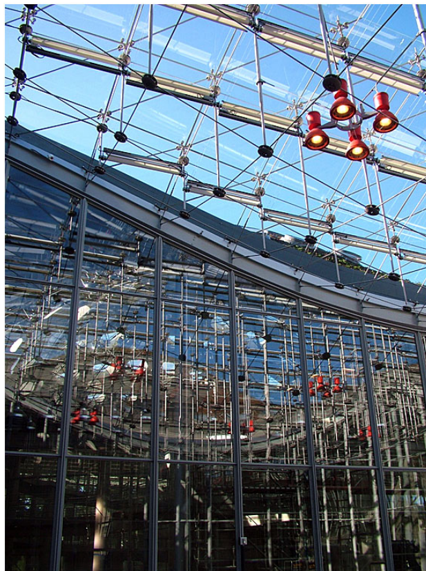
Figure 4.23. View of the Skylight, California Academy of Sciences ( http://philipsgardenblog.com/___onclick_uploads/2008/10/academy03.jpg , July 2010)
