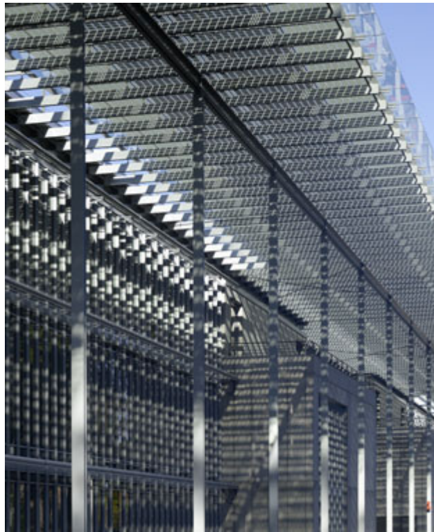
Figure 4.13. Glass Canopy, California Academy of Sciences ( http://www.arcspace.com/architects/piano/cas/academy_of_science_10.jpg , July 2010)
