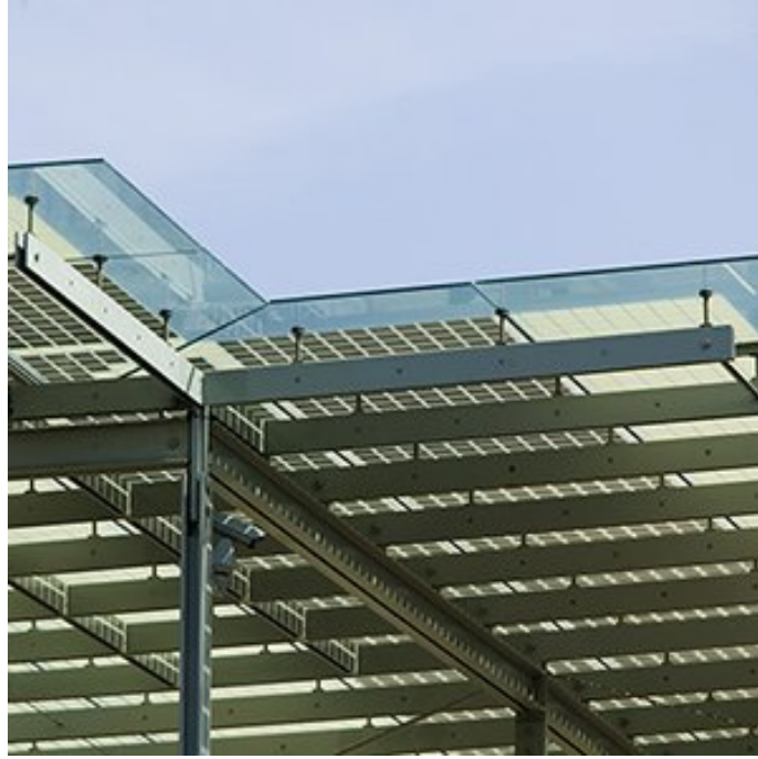
Figure 4.14. Photovoltaics on Glass Canopy, California Academy of Sciences ( http://3.bp.blogspot.com/_0zKcKumK5as/SHVWzJILNgl/AAAAAAAAAFA/KDxPpO52dgY/s400/25722e80-bf22-49ac-94a8-f938d5ef199f.Large.jpg , July 2010)
