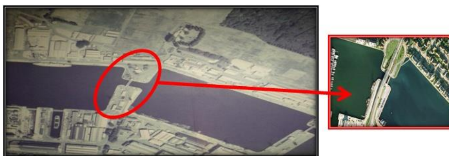
Figure 2. The St Marys Island Bridge previous (left) and recent view (right) [13]
