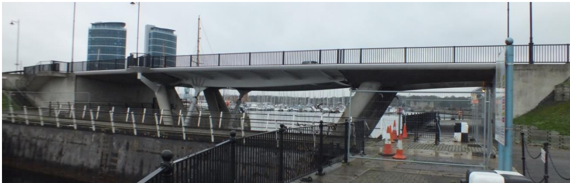
Figure 3. HMS Chatham Bridge [14]
