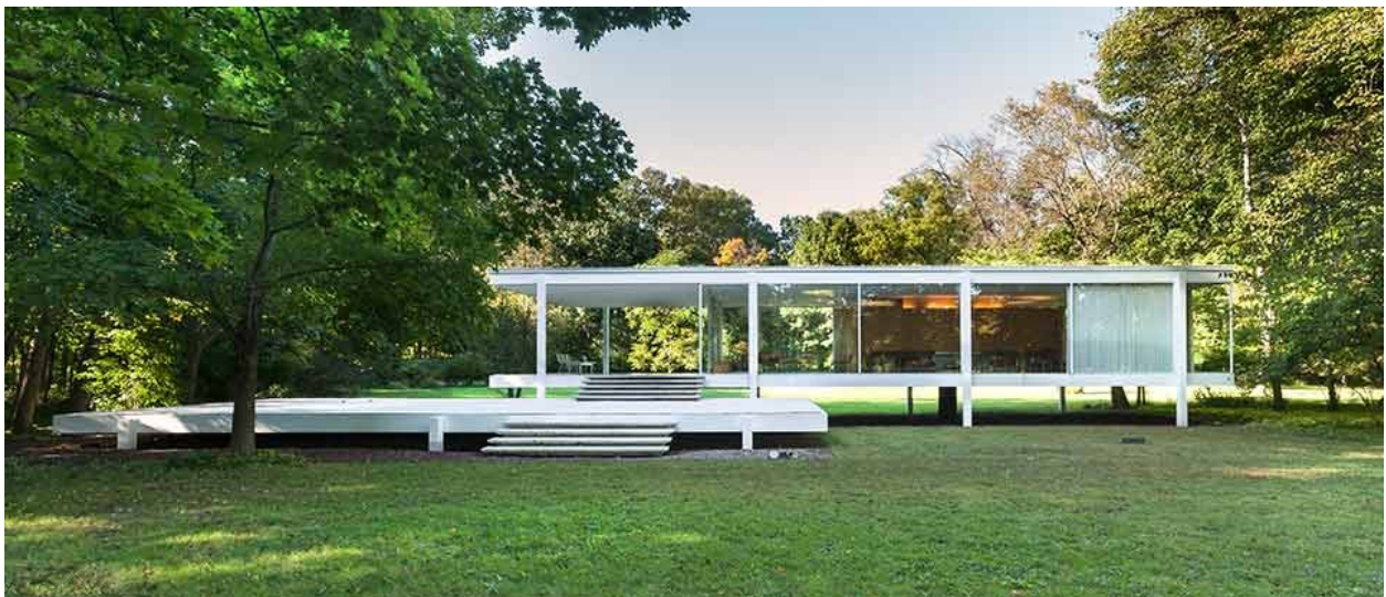
Figure 3.4. Farnsworth House by Mies van der Rohe, Plano, IL, USA. (Source: https://farnsworthhouse.org/ ).
