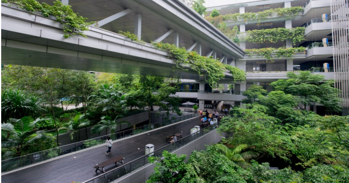
Figure 3.6. Khoo Teck Puat Hospital (Yishun, Singapore). (Source: https://gbdmagazine.com/2018/singapore-hospital ).
