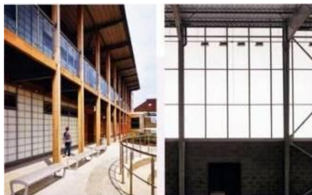
Figure 64, 65 Aerogel filled panel surface in school extension building in London (2005) (Leydecker 133)
