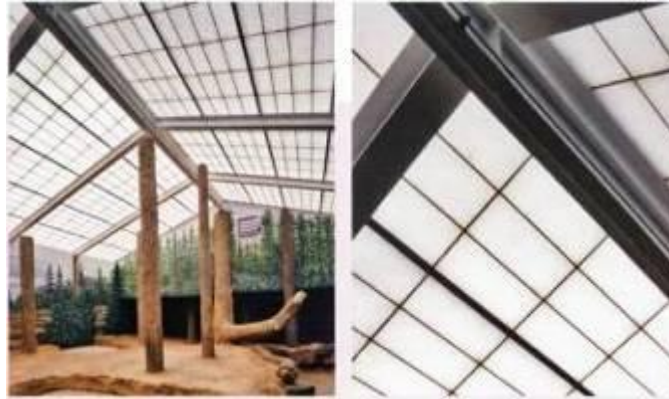
Figure 62, 63 Glass roof of The Florence Mile Borchert Big Cat County building (2005) (Leydecker 132)
