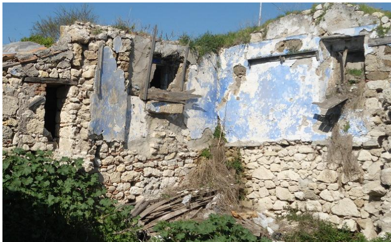
Figure 5.5 Interior Walls in Alaçatı shot taken by Author 2012
