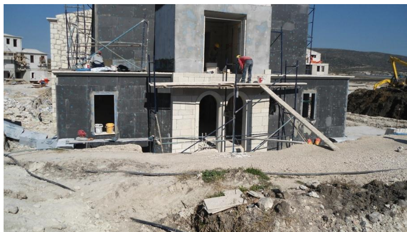
Figure 3.14 Port Alaçatı Construction, photo taken by the Author, April 2012
