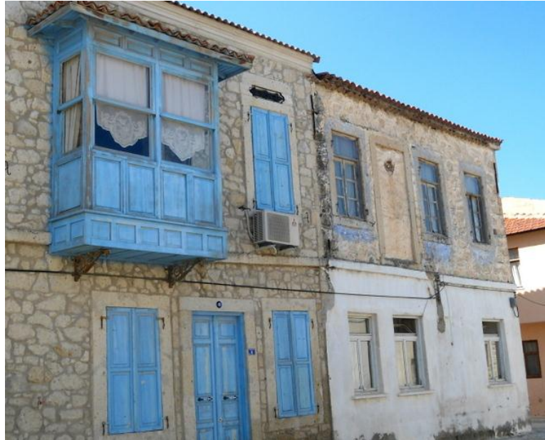
Figure 5.4 Exterior Walls in Alaçatı shot taken by Author 2012
