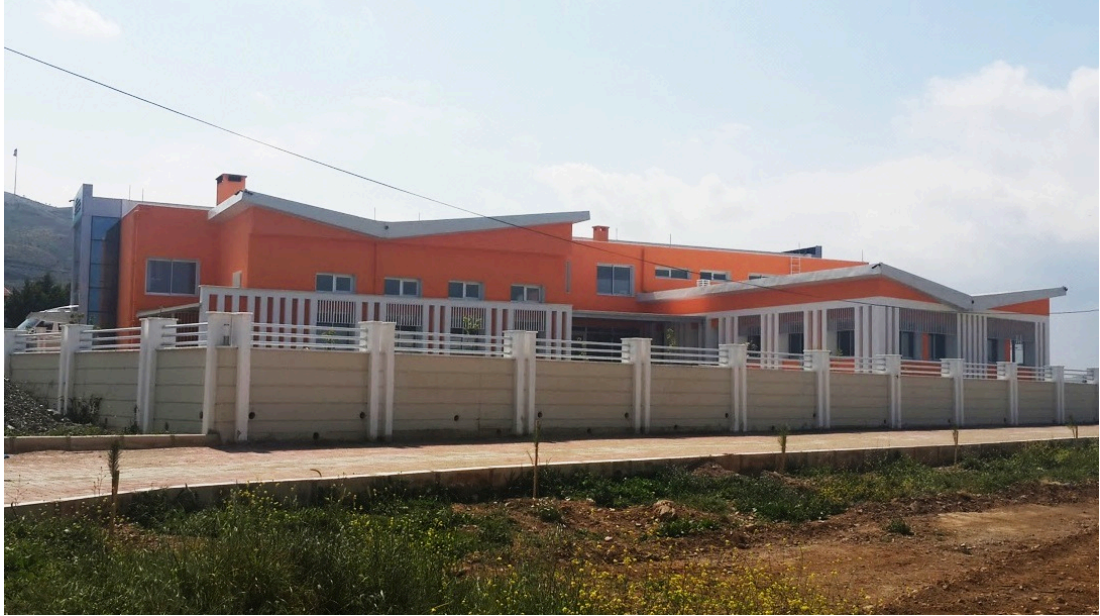
Fig. 4.1 The building of Güzelbahçe Special Education, Application, and Vocational Training Center
