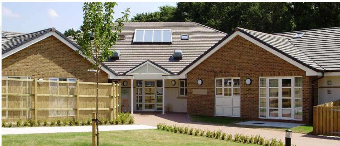
Figure 14. View of Ravenswood residence
