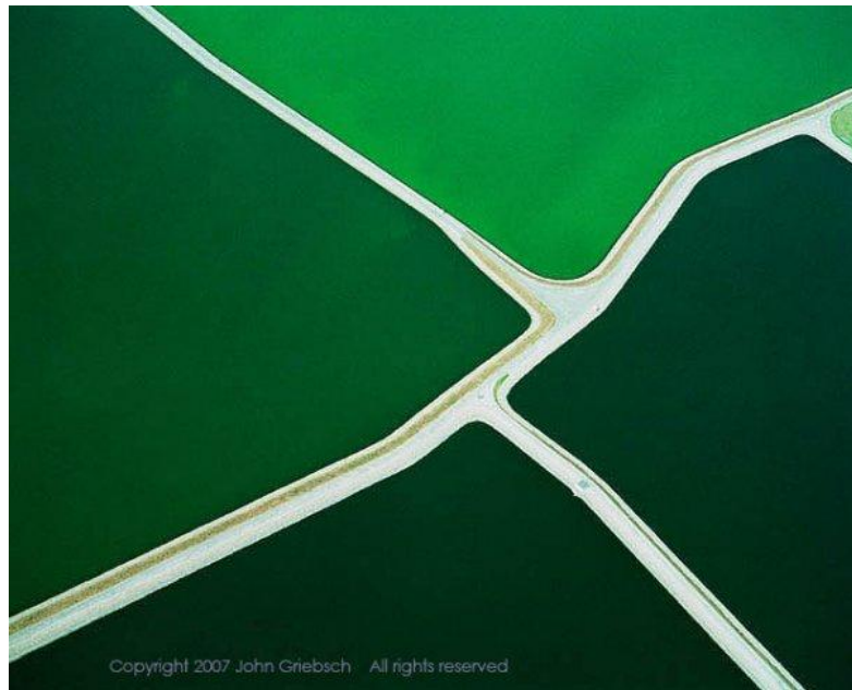
Figure 4.15: Five Treatment Ponds, Batavia, NY
