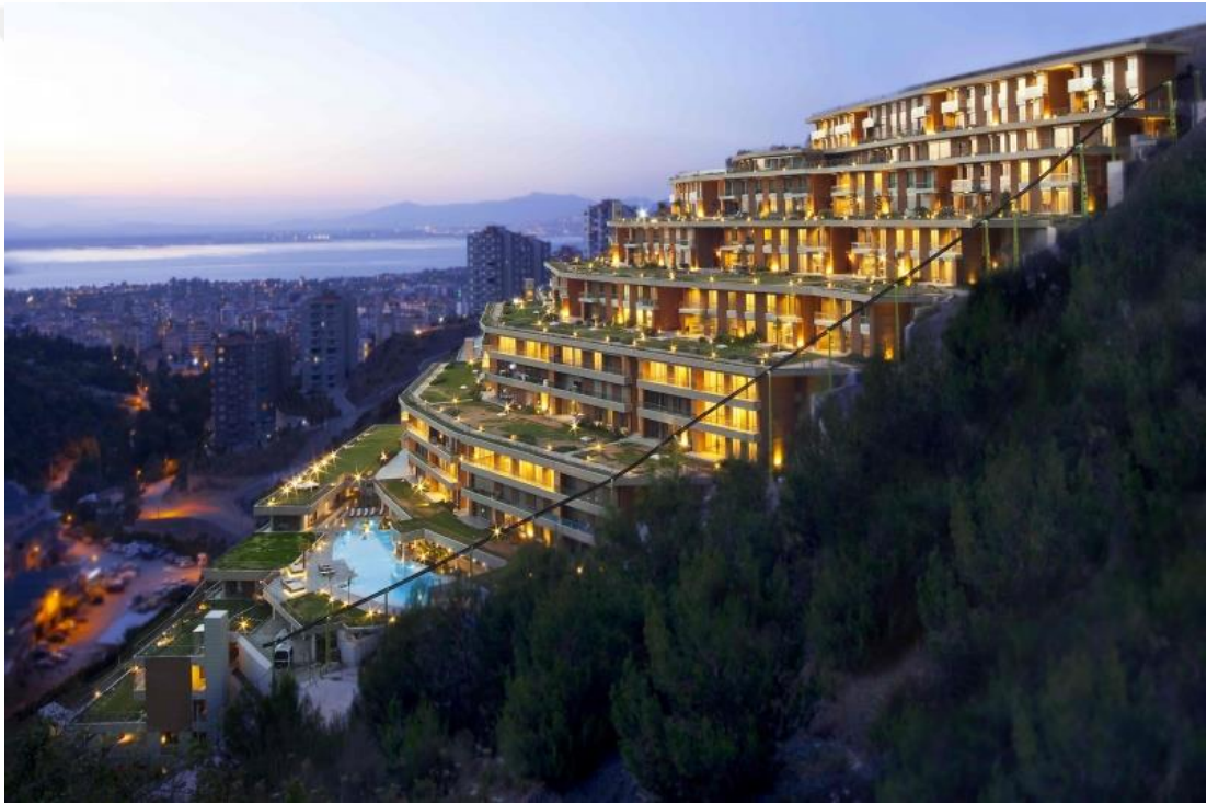
Figure 29. Asma Bahçeler Residence. Architects: Tanyer İnşaat. İzmir.
