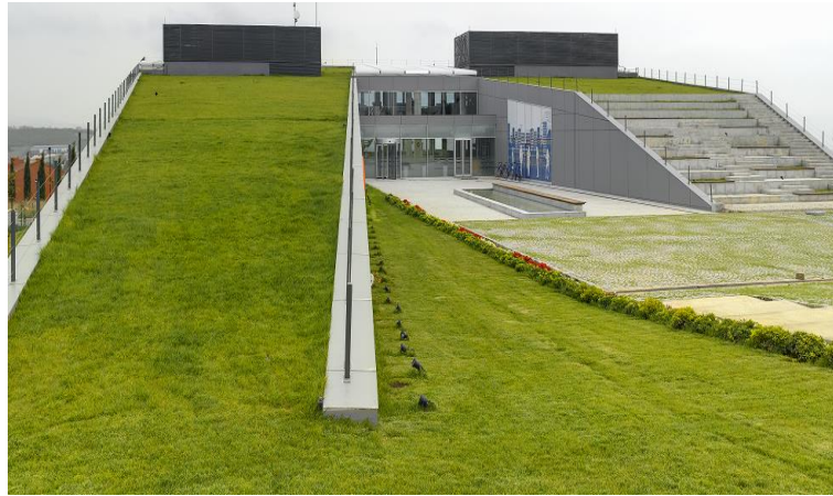
Figure 21. Green roof of Turkcell AR-GE Building / İstanbul
