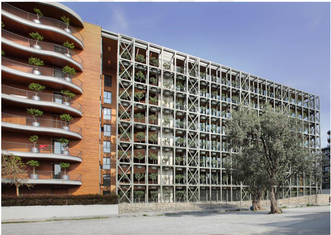
Figure 28. Folkart Narlıdere Residence. Architect: Emre Arolat. İzmir.
