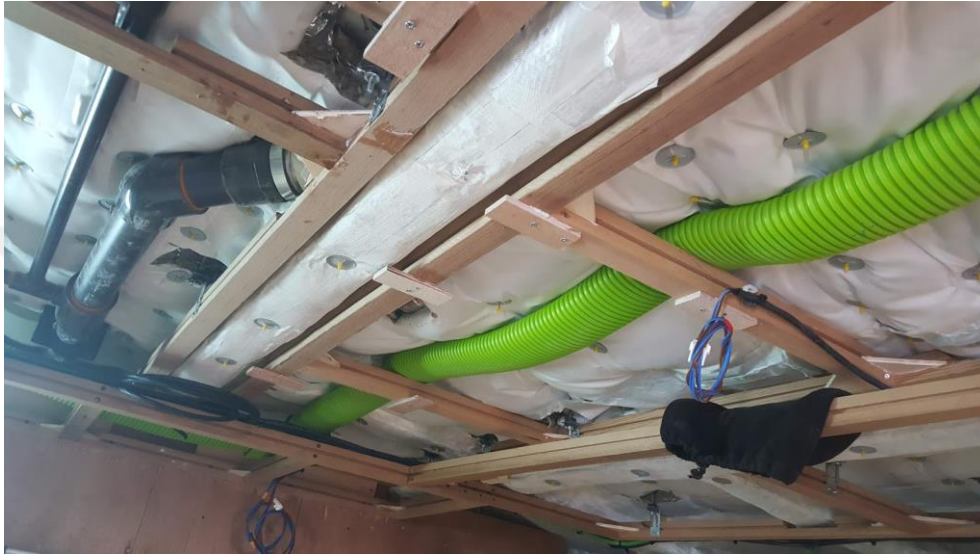
Figure 43. Piping System on the Ceiling Part of a Motor Yacht
