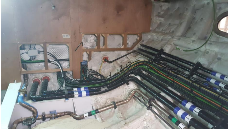
Figure 32. Interior Frames to Divide Areas and Cover the Necessary Cable Units
