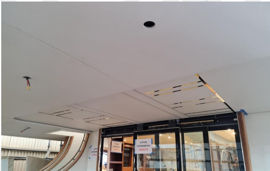
Figure 17. Exterior Lightning Application
